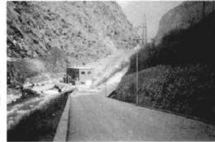
The Bhote Koshi Hydroelectric Project site
